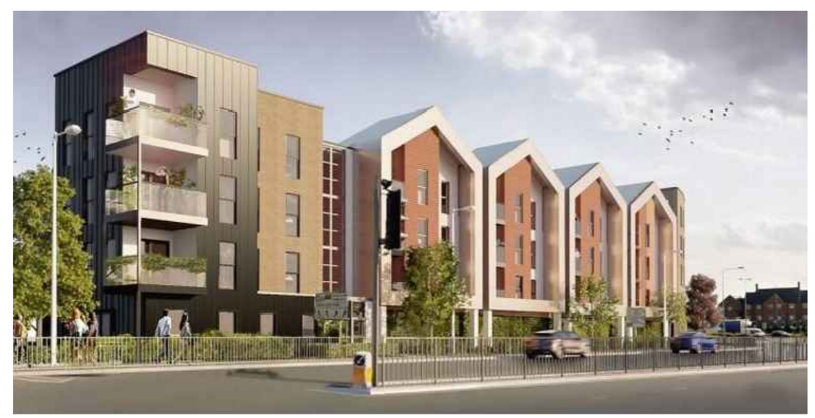
McCarthy Stone development in chelmsford with projecting gables.
