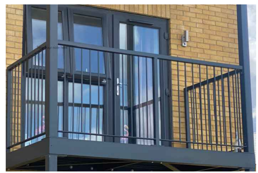
Steel balconies with vertical railings set between projecting gables or with corner posts dependant on location.
